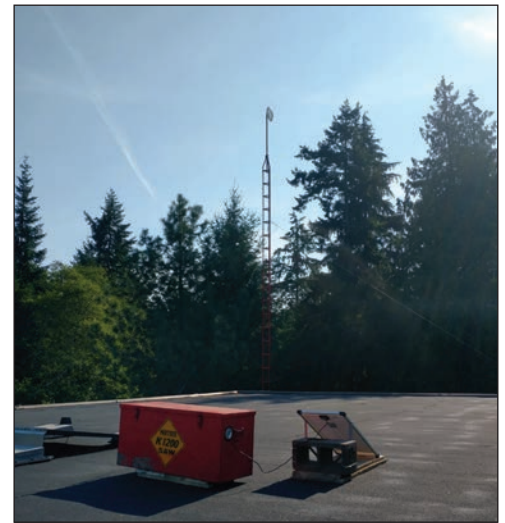
Gabriola AREDN Node temporary first set up on the roof with 40 watt solar panel and 90 Ah 12volts.
